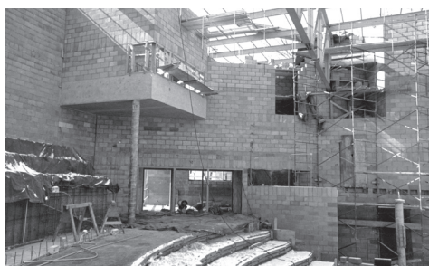
Photo of the Marx Theatre construction.
